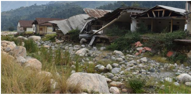
Section of houses which were destroyed by river Nyamwamba floods in Kasese district
